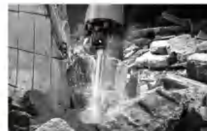
[ 墙体强劲破拆 ]
